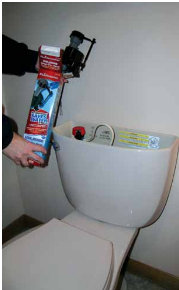
A simple and inexpensive refit program involves kits to repair leaks that are estimated to affect 25 percent of all toilets.
